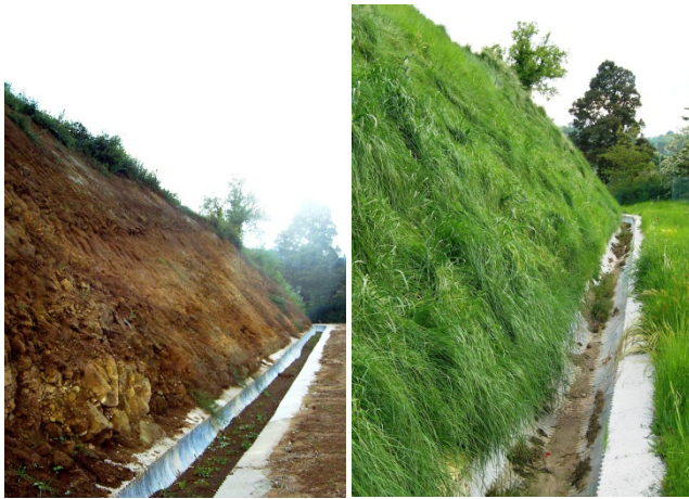
a) clogged drains
