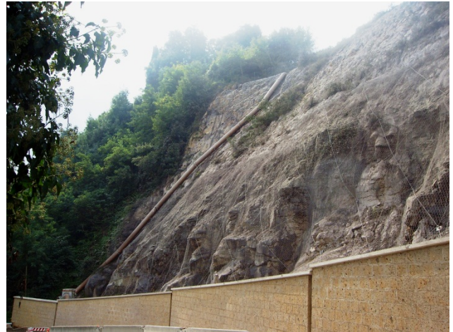
Figure 5a Orvieto (Terni, central Italy), road “SP111 della Badia” Situation of the slope in December 2004, before intervention
